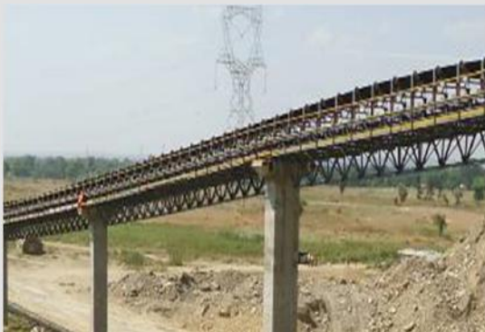
Overland Belt Conveyor
